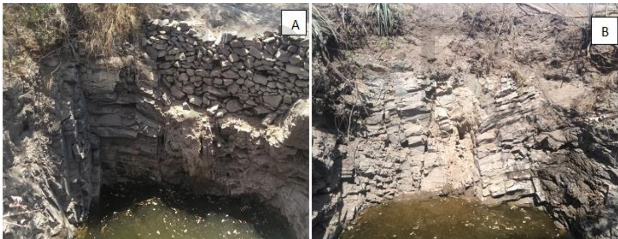
Fig. 6 a) Transverse joints in dyke showing inclined joints. b) Horizontal joints in dyke and also possess nearly 0.6 meter thick intrusion of calcareous material.
